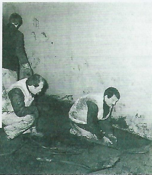
Scooping out earth to enable air bags to be placed under trailer.
