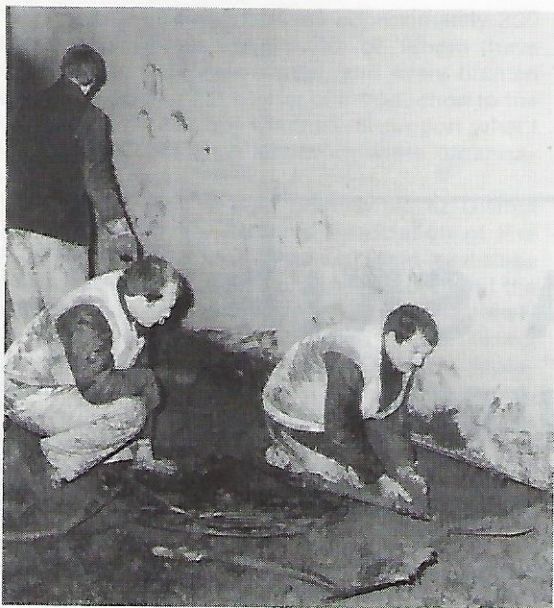
Scooping out earth to enable air bags to be placed under trailer.
