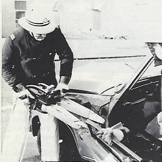
Removing door with the jaws
