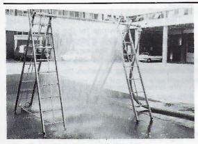
It was while I was taking part in the recruits Pass Out Drills that I had the idea to get a damaged pole from a 135 ladder, fit a male instantanious coupling one end and a female at the other. As luck would have it, the 45mm coupling was a close
