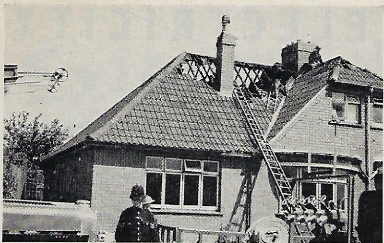
THE RESULTS OF A SHORT CIRCUIT IN THE ELECTRICAL WIRING
